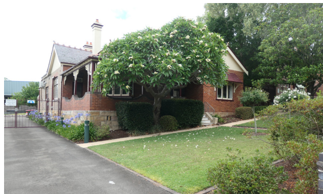
Figure 2.4 Rose Cottage at 31 Bancroft Avenue, exuding characteristic features of the Federation style such as the face brick, street facing gable, sandstone base and wrap around verandah
